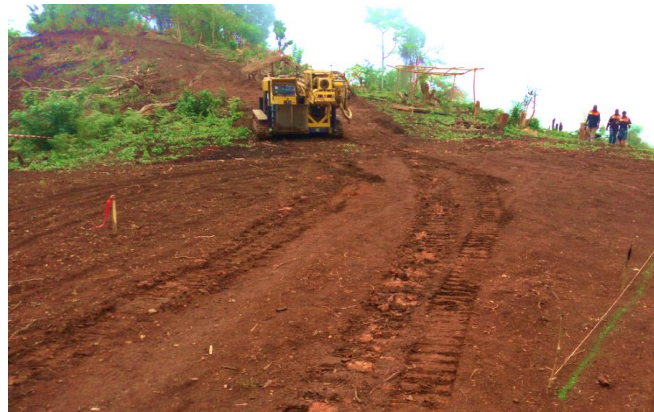
Access road to the project site
